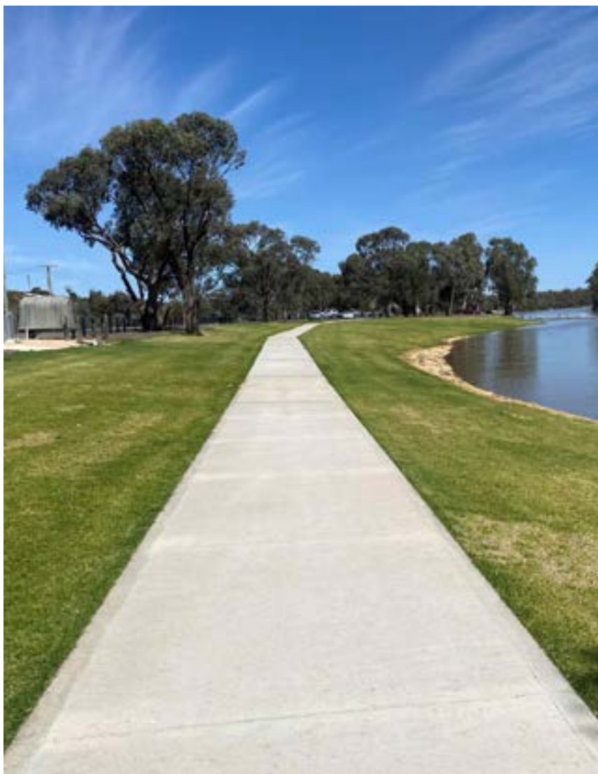
New walkway and viewing platform at Loxton riverfront
