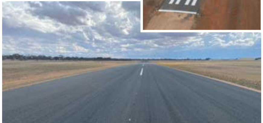
Re-seal of Loxton and Waikerie airstrips
