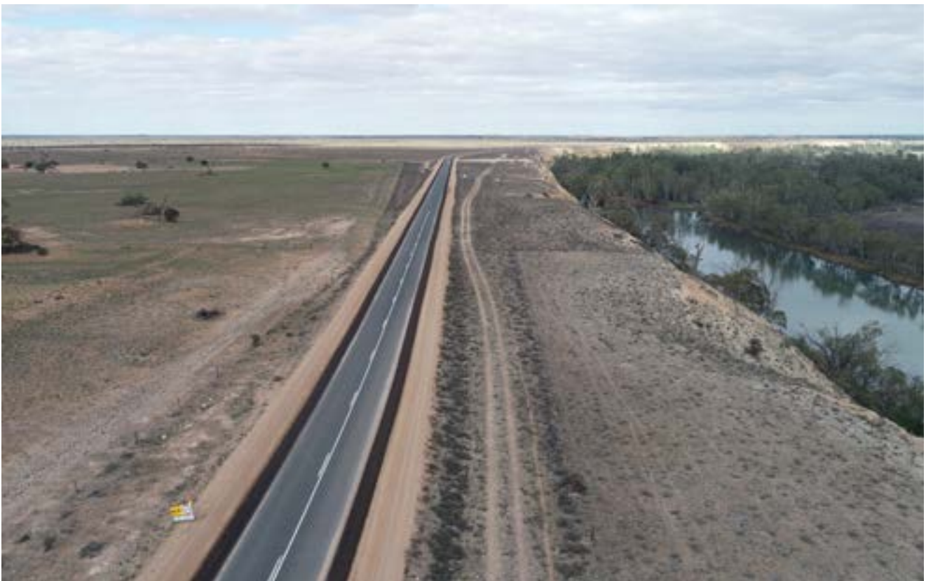
Murbko Road verge widening and resealing
