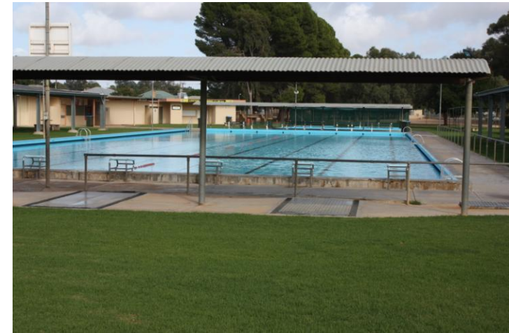
The pool is the only 8 lane outdoor 50m pool in the Riverlands
