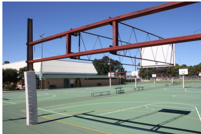
Courts are dual use marked for both basketball (summer) and netball (winter) with retractable basketball and removable netball rings
