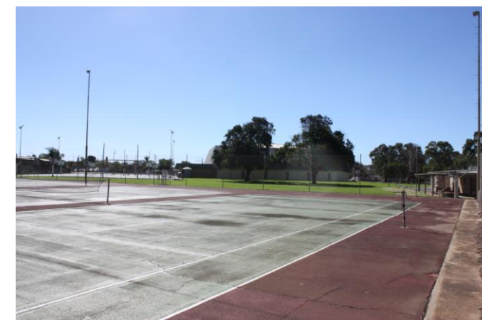
Six disused tennis courts provide opportunity for use for netball development but are in need of resurfacing.
