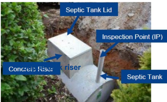
Diagram showing the different parts of a septic tank.
