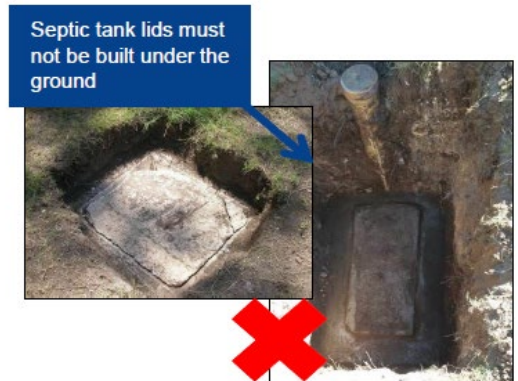
Septic tank lid ground level for maintenance and pumping out
